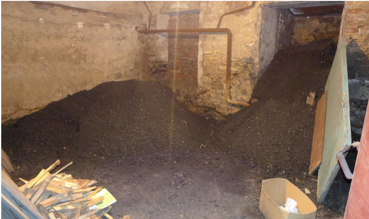
Coal storage bunker
